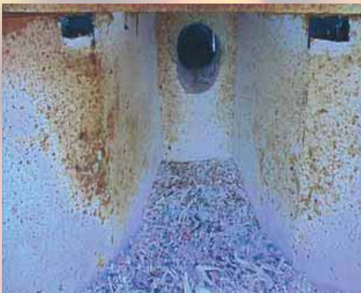
Internal view of primary chamber
